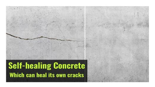
Bio-mineralization techniques give promising results in sealing the micro-cracks in concrete. The freshly composed micro-cracks can be sealed up by perpetual hydration process in concrete.
